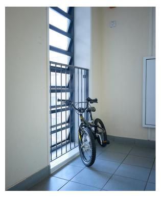
LAMILUX successfully installed the 28 TGL louvre windows, improving ventilation and the overall environmental efficiency of Dominion House. The careful planning, delivery, and installation processes ensured that the project was completed smoothly, with minimal disruption and maximum effectiveness and all materials were disposed of using the supplied skip.
