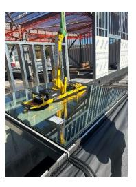
A total of seven mono-pitch rooflights have been installed, of which two feature fire-resistant glazing designed to provide fire protection capable of enduring flames for up to 60 minutes. The other five rooflights are fitted with double-glazed Easy Care Glass that includes a self-cleaning effect (Bioclean).
