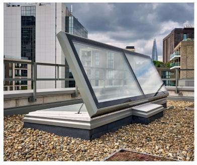
LAMILUX provided two Access Swings with left-hand openings and two with righthand openings to guarantee accessibility to the roof space.
